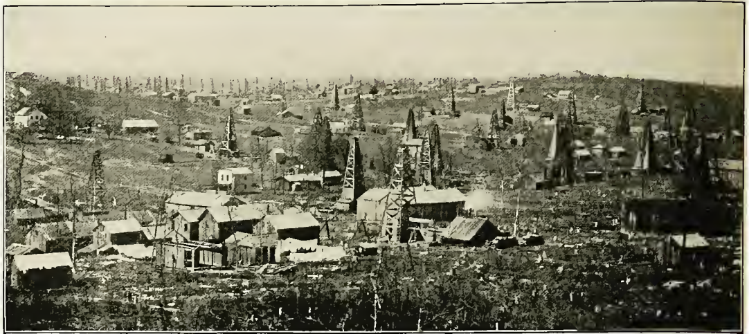
FIG. 144. — A view in the oil fields of western Pennsylvania. Each of these small towers, or derricks, stands over an oil well. The derricks were used in boring the wells.
